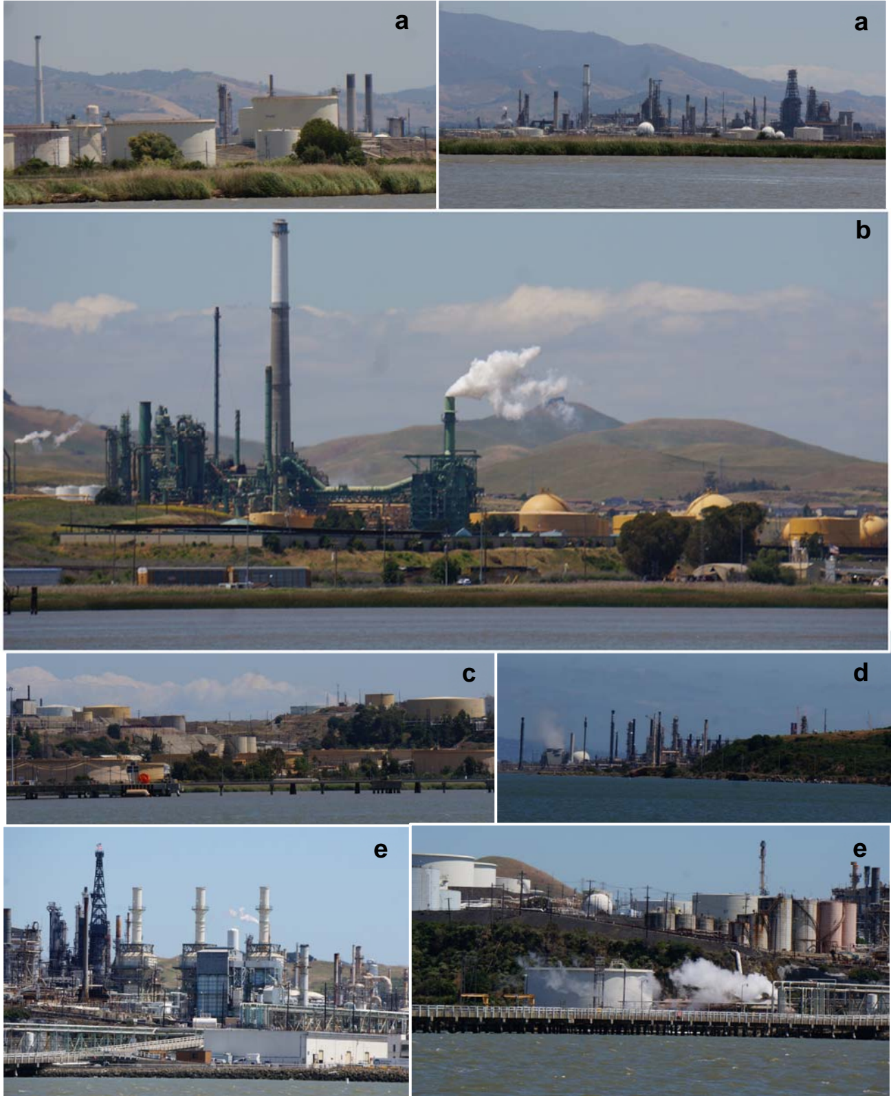
Figure 11. San Francisco Bay Area TFS Hub Refineries. a) Andeavor (ex-Tesoro) refinery. b) Valero refinery. c) Chevron refinery. d) Shell refinery. e) Phillips 66 refinery.
